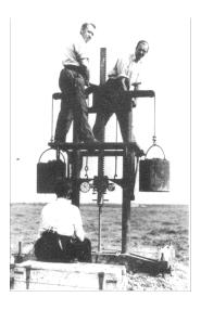
Figure 4 Early Dutch mechanical cone (after Delft Geotechnics)
